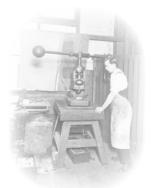
Die sinking the individual lead matrices used in the form
