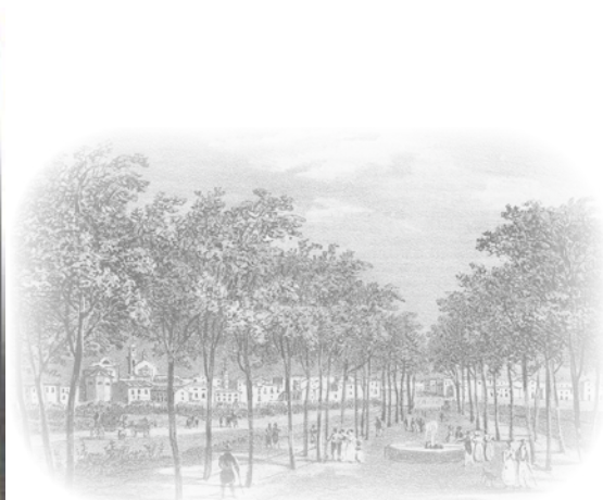
View of Foggia
