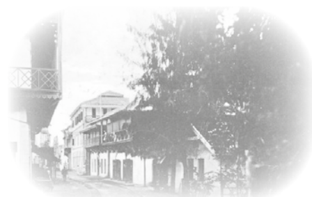
Imperial British East Africa laid railroad tracks through Mombasa
