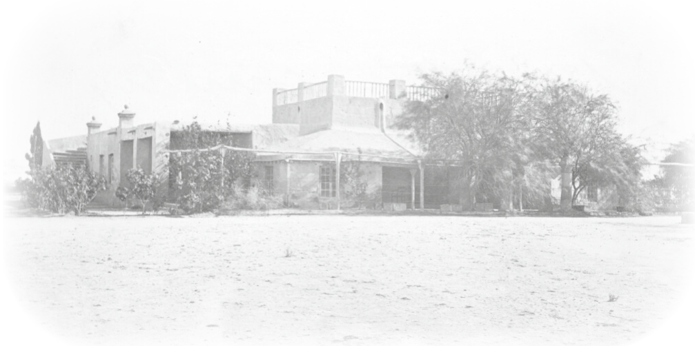
British resident's country house in Bushire
