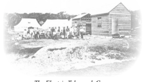
The Electric Telegraph Camp laying the cable
