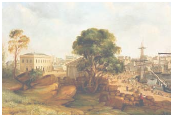
Custom House and Circular Wharf in Sydney
