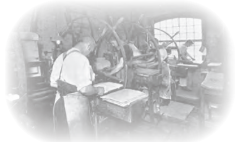
Perkins Bacon printing presses used for the stamps
