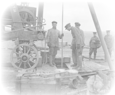
Royal Engineers boring a well to supply water to the army
