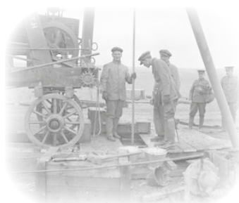
Royal Engineers boring a well for the British Army in Salonica
