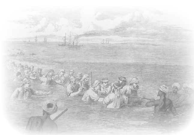
Installation of the cable for the telegraph line in the shallow waters of the Persian Gulf
