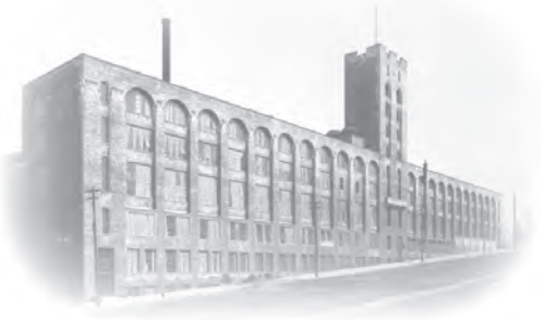
American Bank Note Company Printing Plant
