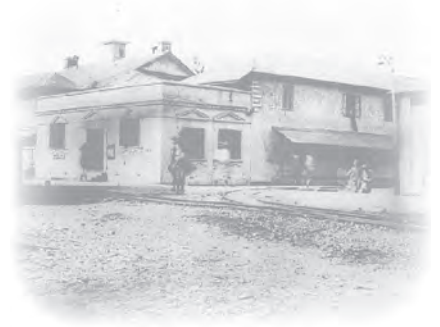
Post Office in Lagos
